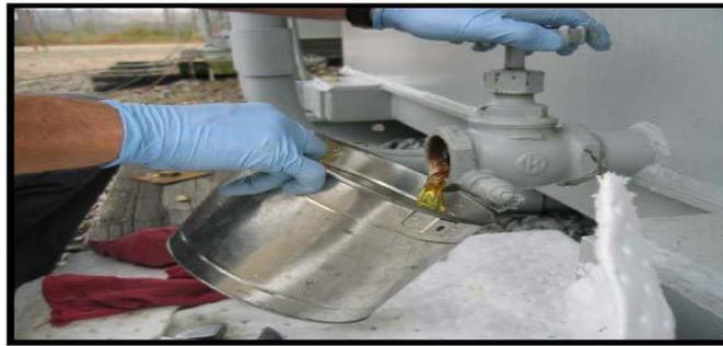
**Figure 3:** Discharge of oil at the lowest point of transformer
