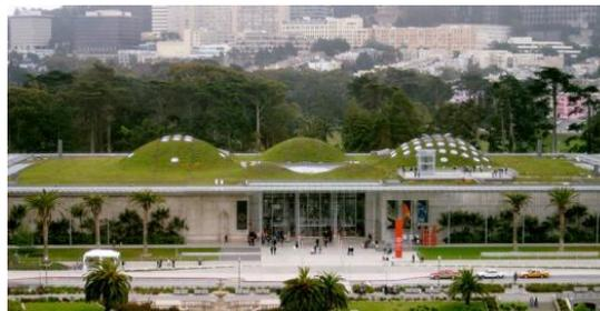
**Figure 6.** Semi-intensive green roof
