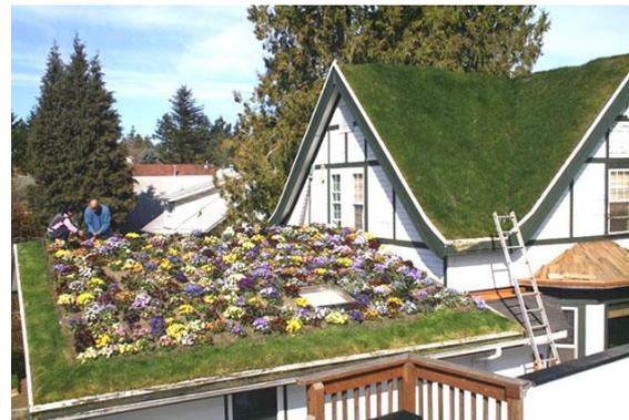
**Figure 3.** Extensive roof with drainage system: 1) extensive lawn – vegetation; 2) soil layer 80-100 mm thick; 3) separation/filtration layer; 4) drainage layer; 5) fabric (e.g. polypropylene) 110-140 g/m<sup>2</sup>; 6) insulation material; 7) bituminous waterproofing sheet; 8) concrete ceiling
