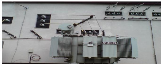
**Figure 1:** Transformer connected to the electrical grid in substation 35/10 kV [1]
