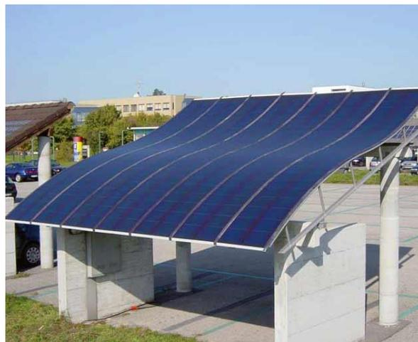
**Figure 2.** Thin Film Solar Panel [11]
