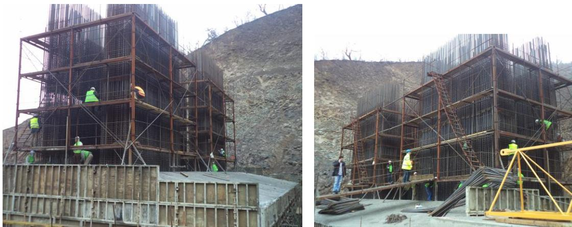
**Figure 2.** Scaffolds and ladders established on the bridge No.5 at Motorway construction Demir Kapija - Smokvica
